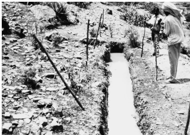
Fig. 3. Sediment collecting trench in the rangeland of Luqmuta at the end of the rainy season.
